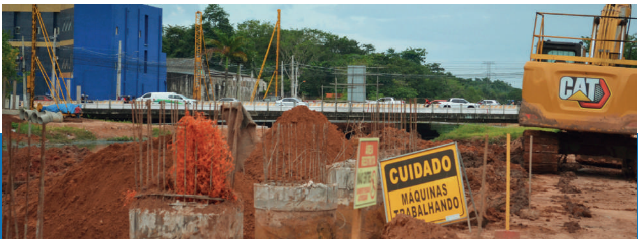
Photo: Construction works in the Igarapé São Joaquim territories, July 2025.
